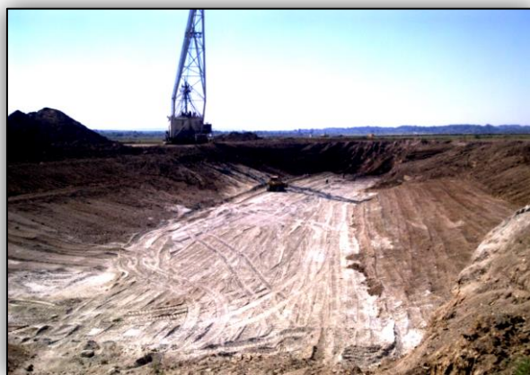
Figure 2. Excavation test sections of the Kolubara River Gorge
