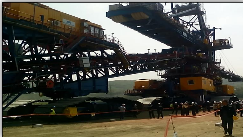
Figure 1. Tray starting at the planned location of the conveyor belt for work, (2016, EPS, Branch RB "Kolubara")
